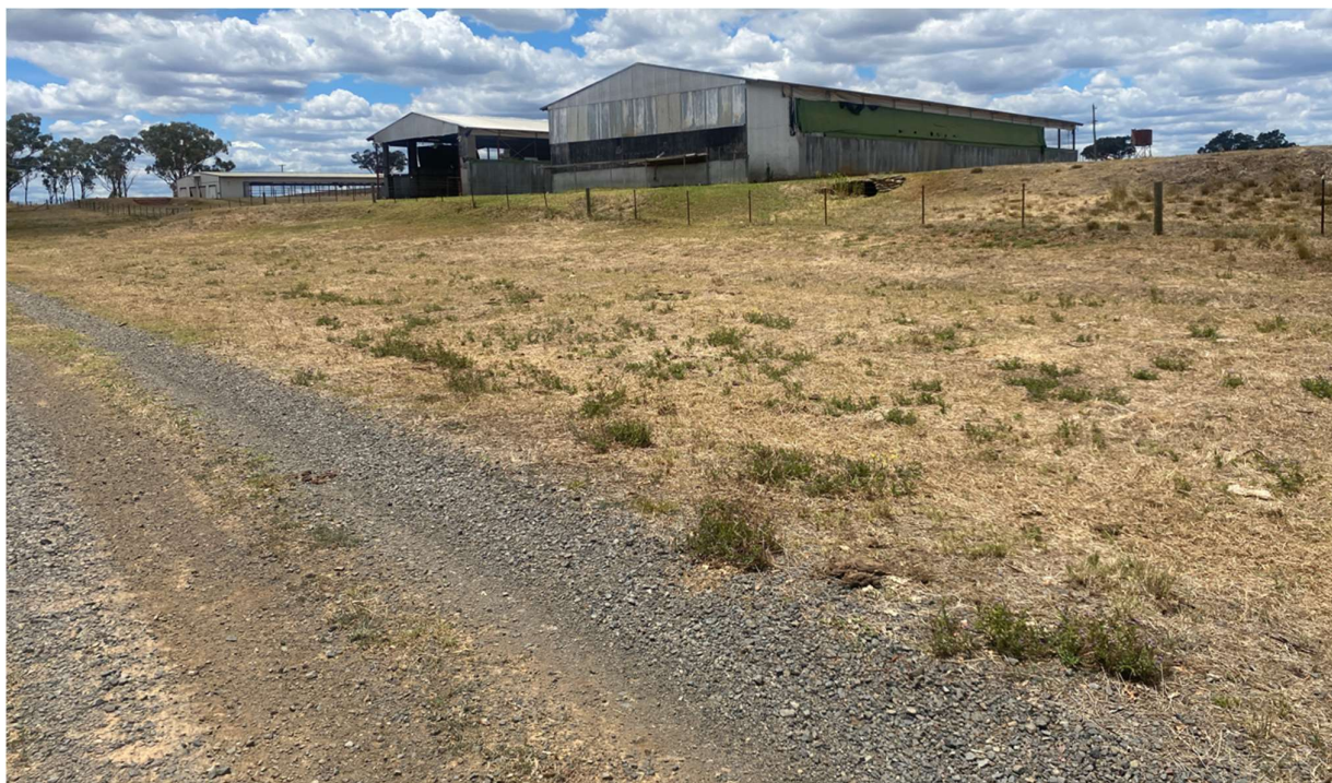
Figure 8: Drainage line from neighbouring decommissioned poultry sheds into subject site – facing north east
